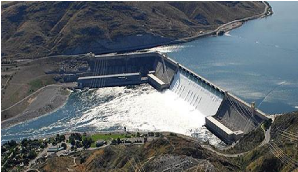
Grand Coulee Dam on the Columbia River
